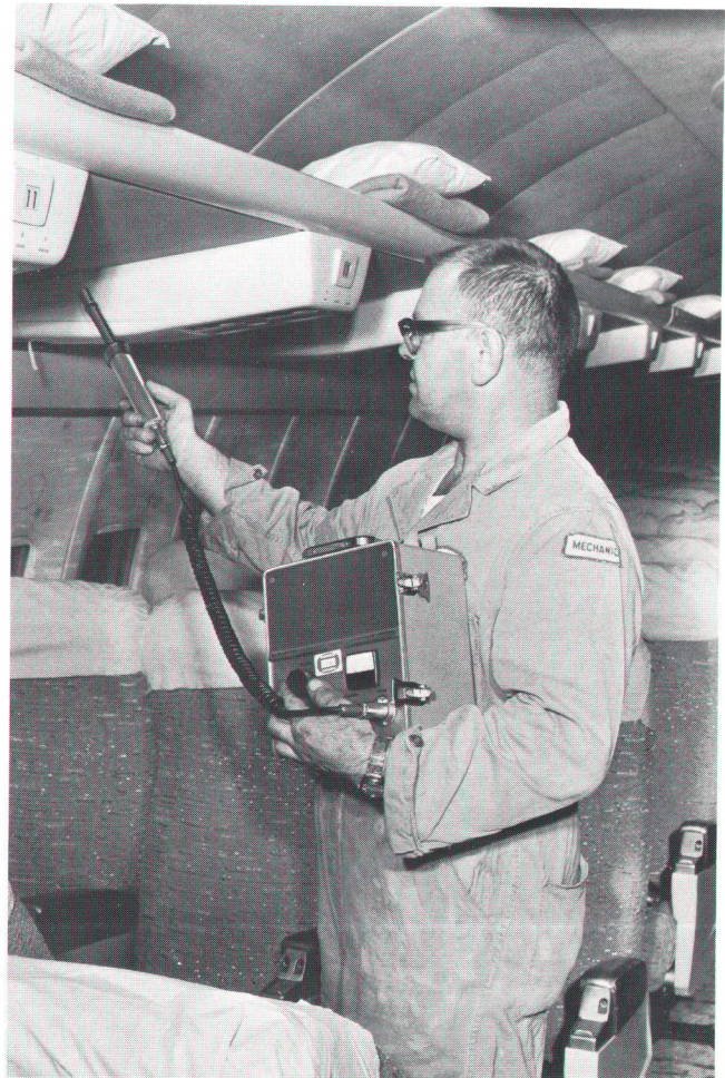
Airline mechanic checks Boeing 720B cabin oxygen system for leaks using -hp- Model 118 Ultrasonic Translator and general-purpose probe with focusing extension.
